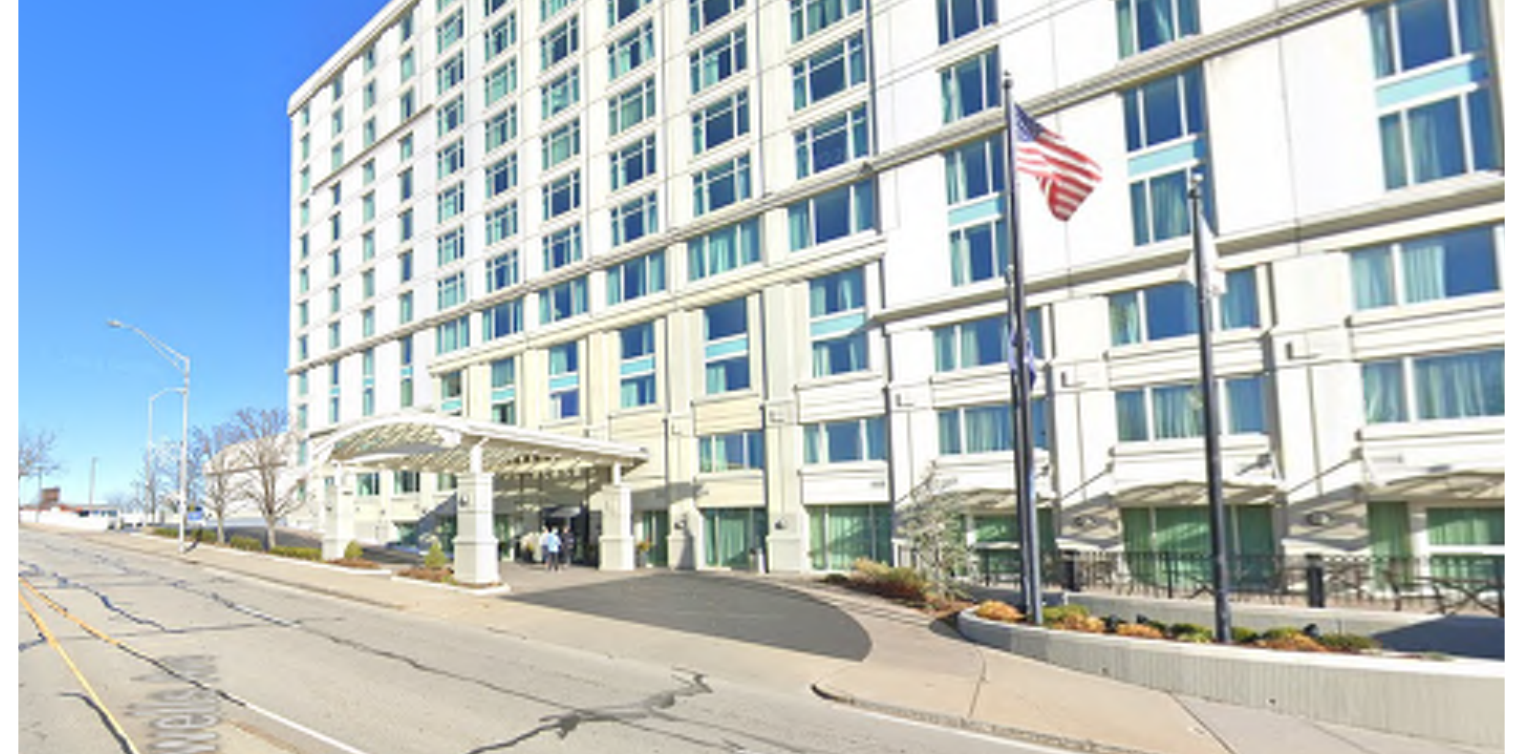
EAST VIEW OF EXISTING HOTEL ENTRANCE
