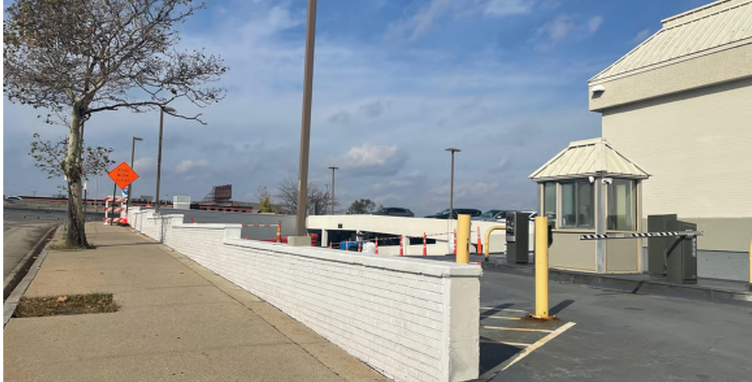
VIEW LOOKING NORTHWEST TOWARDS HIGHWAY RAMP
