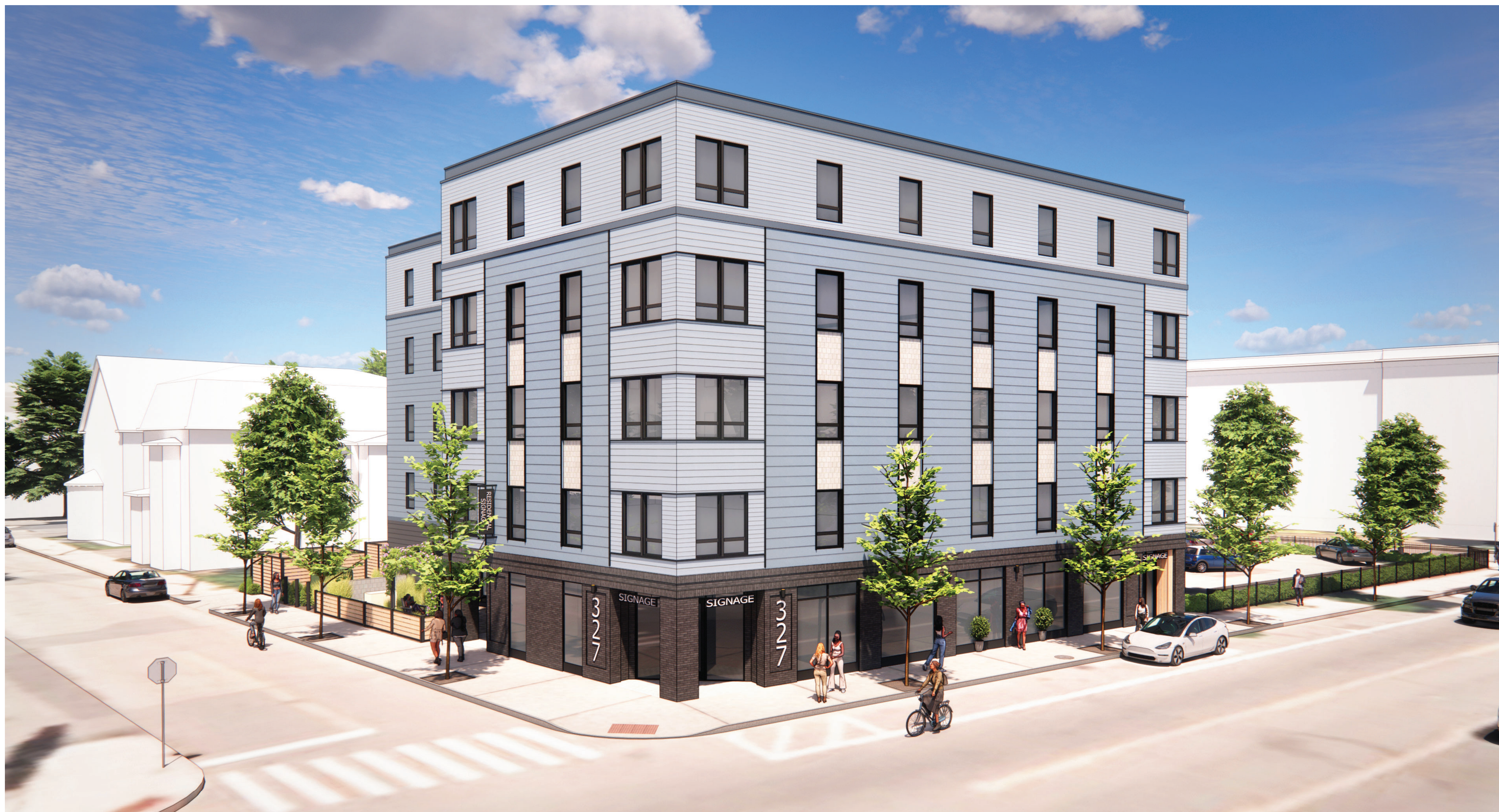
VIEW OF PROPOSED BUILDING FROM ELMWOOD AVE
