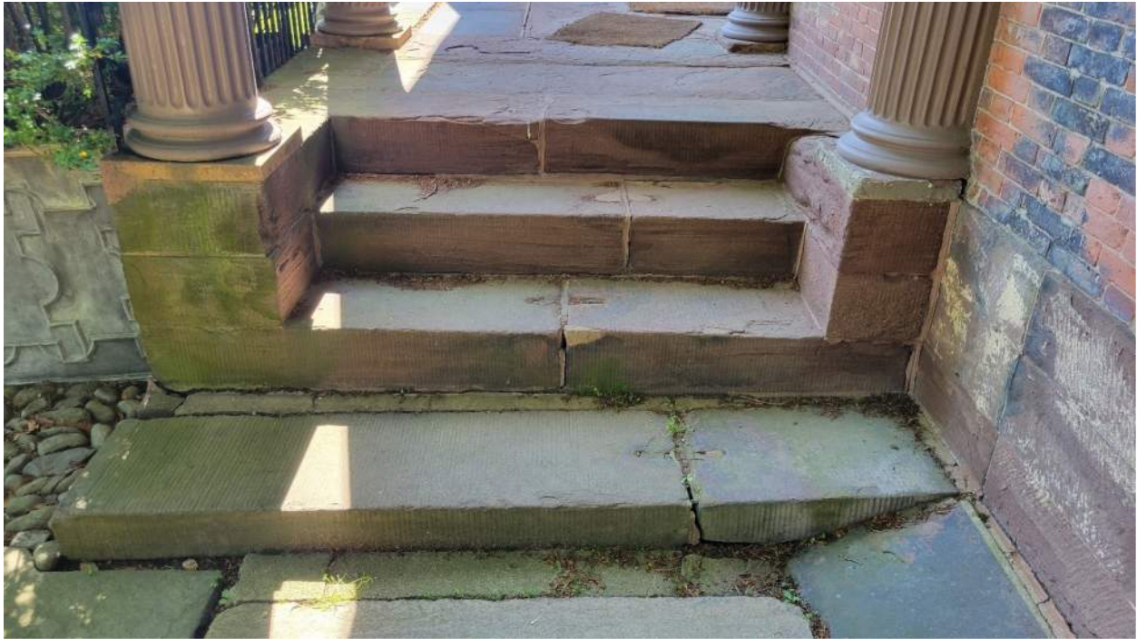
21. Brownstone displacement at front entrance porch
