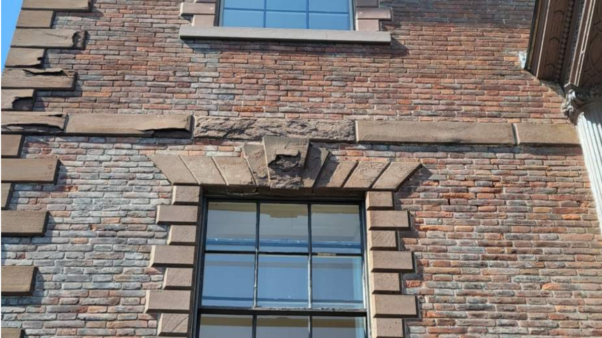
23. Brownstone deterioration at south elevation trim
