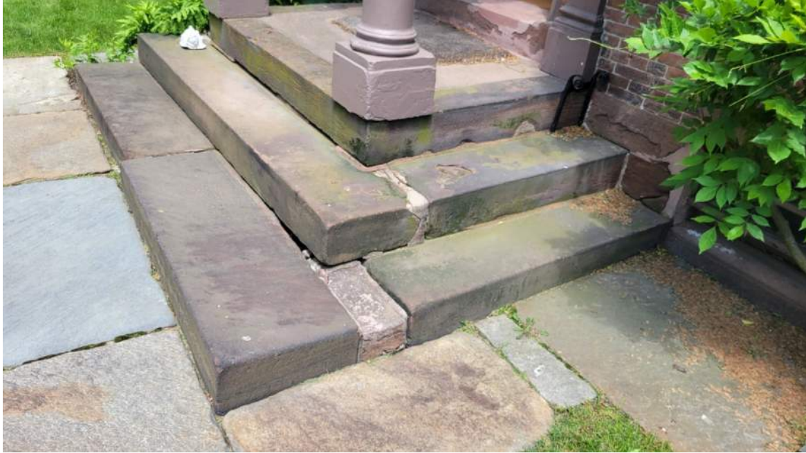
13. Brownstone deterioration and displacement at west portico
