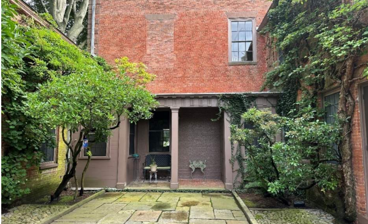
25. Rear (north) porch at main block (note second floor filled-in window to be recreated)
