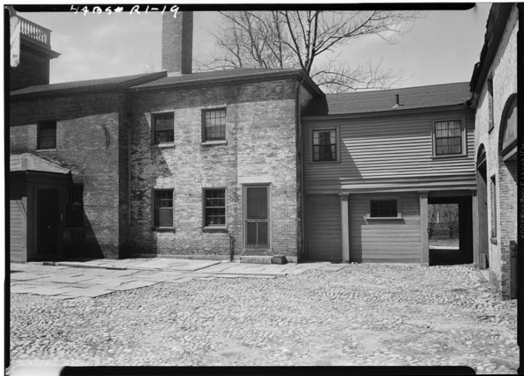
30. 1936 HABS photo of connector (note wood infill just behind columns)
