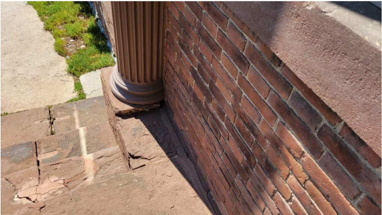
20. Brownstone deterioration at front entrance porch
