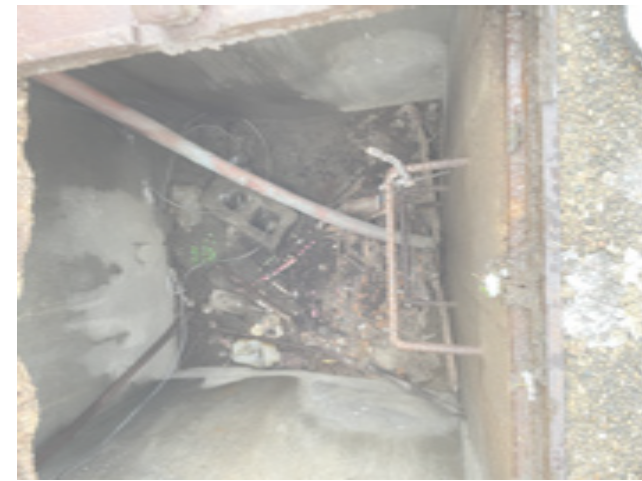
C WATER METER PIT INTERIOR
