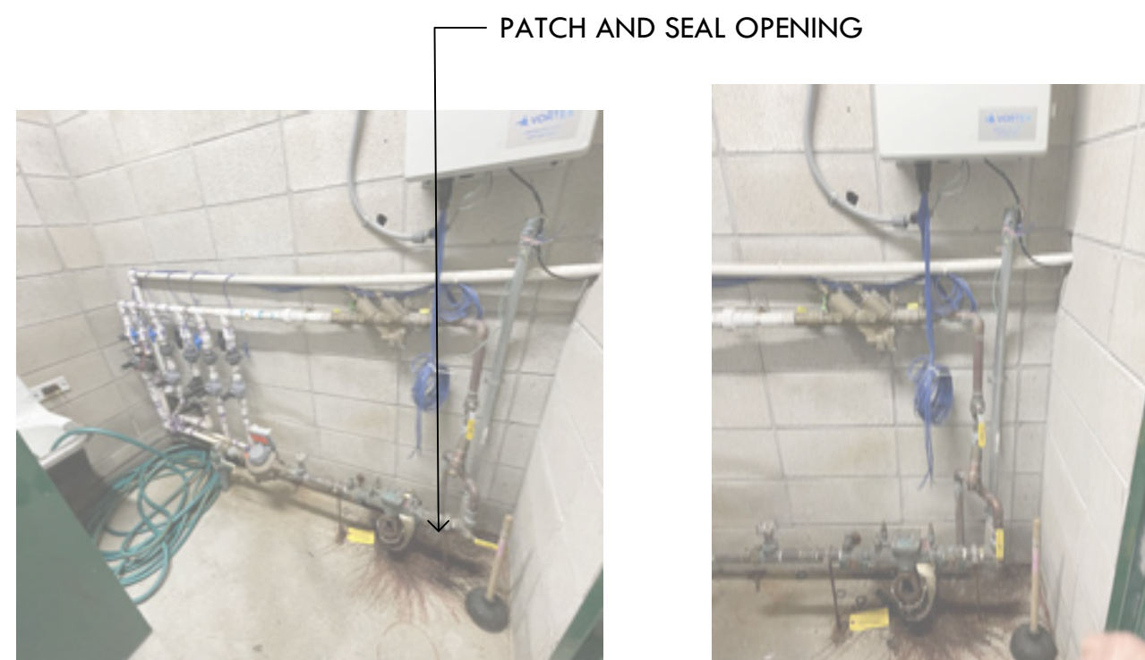
D FACILITIES BUILDING INTERIOR: EX MANIFOLD, BACK FLOW VALVES & CONTROLLER E FACILITIES BUILDING INTERIOR: VORTEX CONTROLLER & POWER ADAPTER
