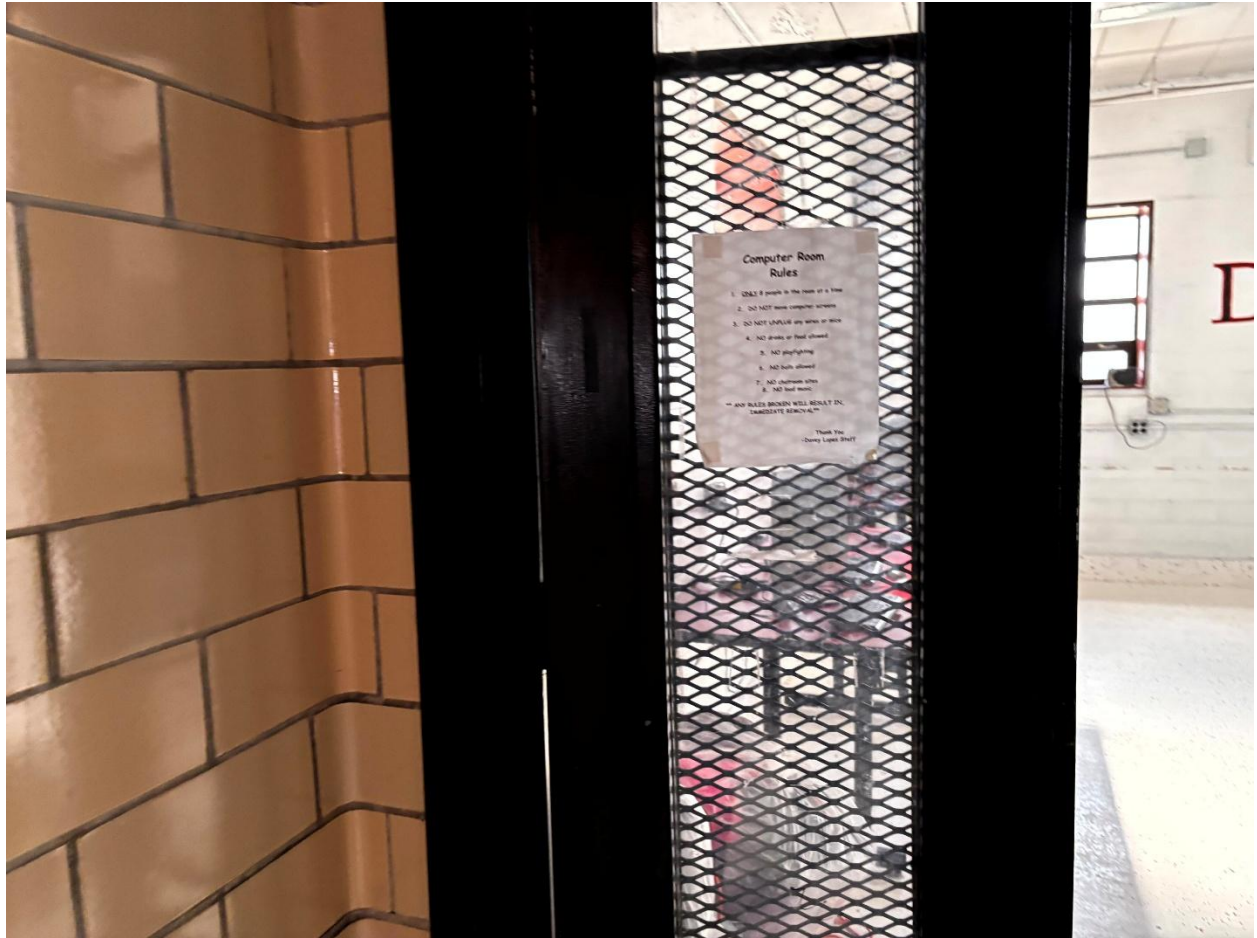
Interior door glaze contains ACM.
