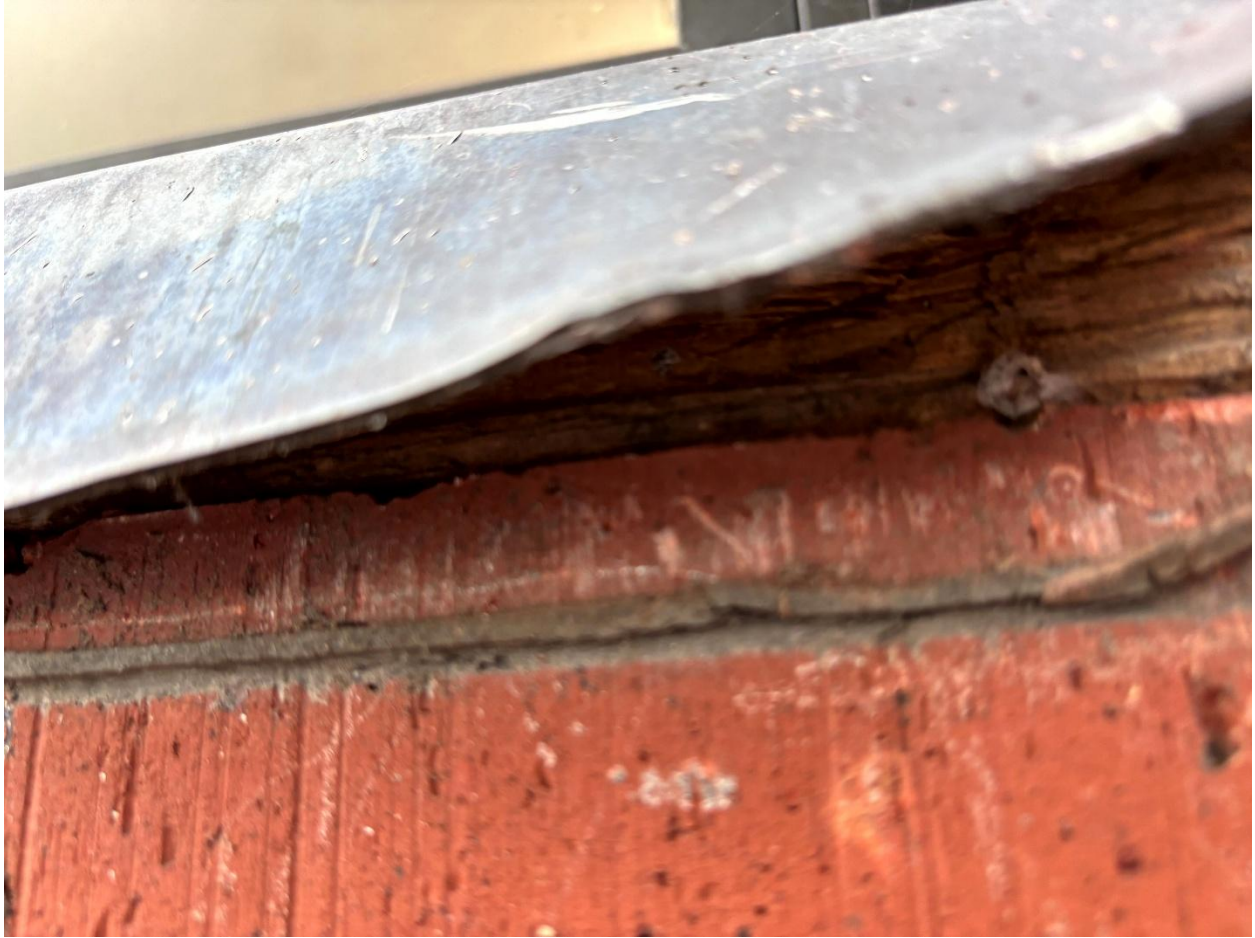
Thin caulk under exterior aluminum window sill contains ACM.
