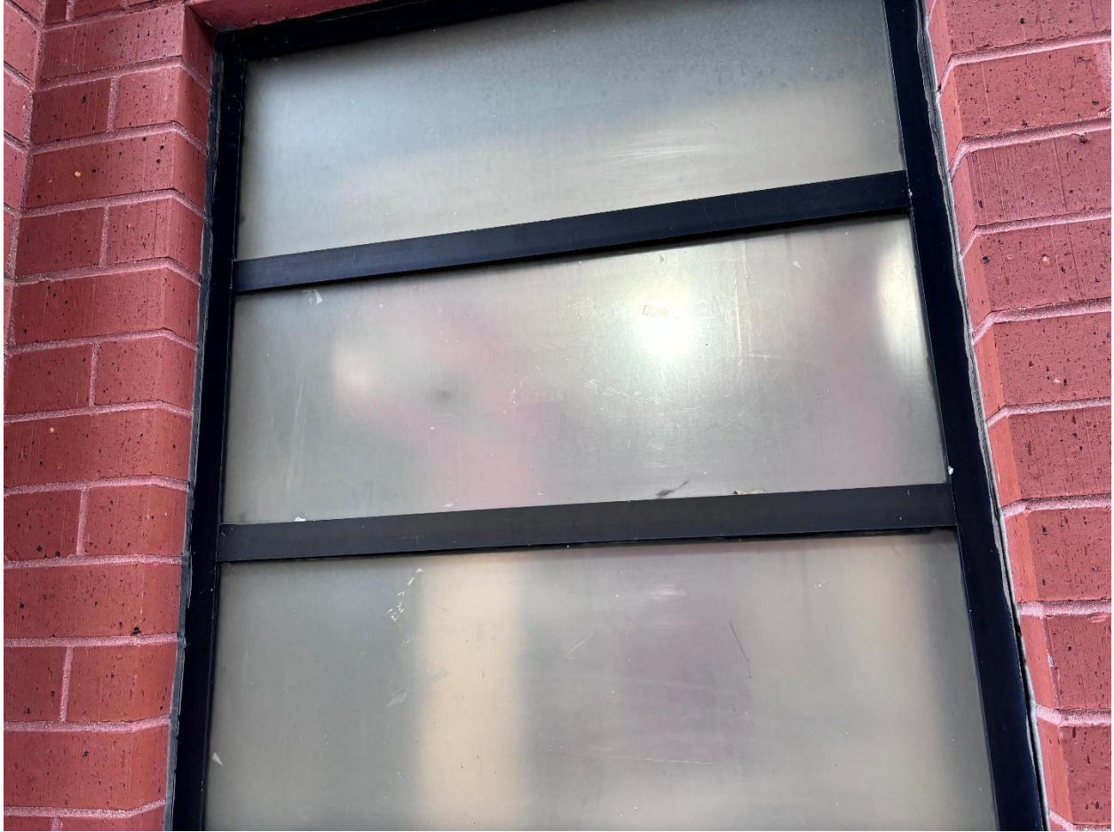
Exterior window caulk and glaze contain ACM.
