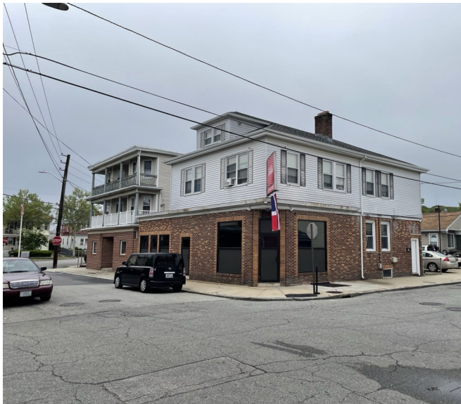
View of the building from Ethan Street
