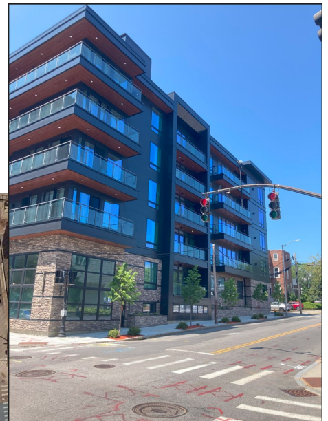
View from Brook Street
