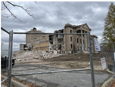
View of building from Princeton Ave
