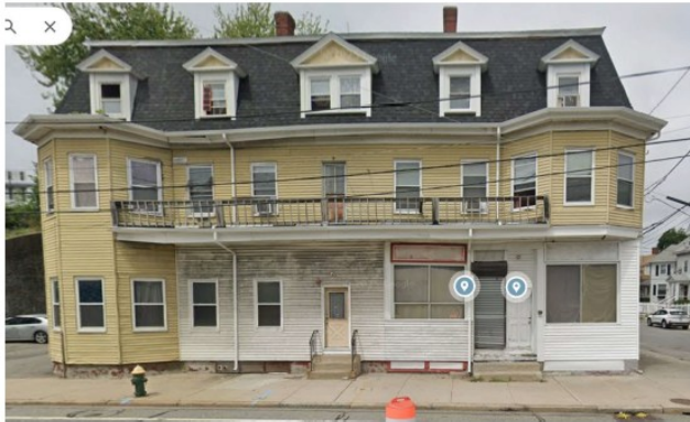
View from Elmwood Ave
