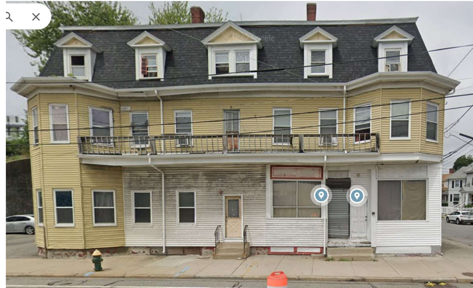
EXISTING FRONT VIEW
