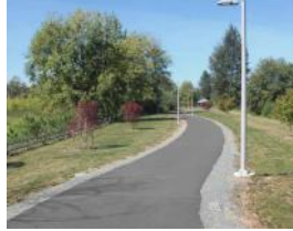
ASPHALT PATH WITH LIGHT POLES
