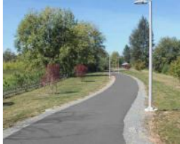
ASPHALT PATH WITH LIGHT POLES
