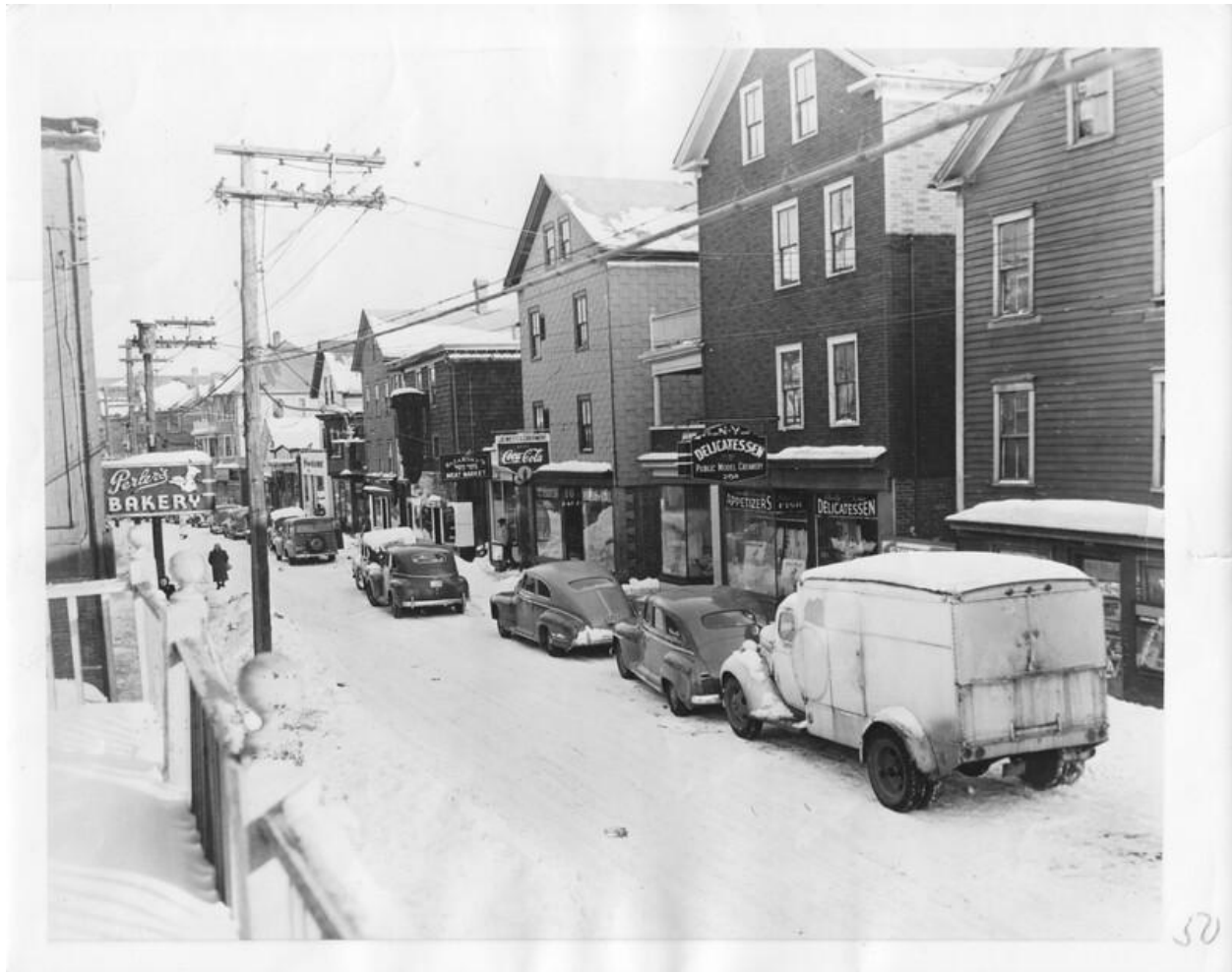
Figure I: Willard Avenue Before Redevelopment, 1947
