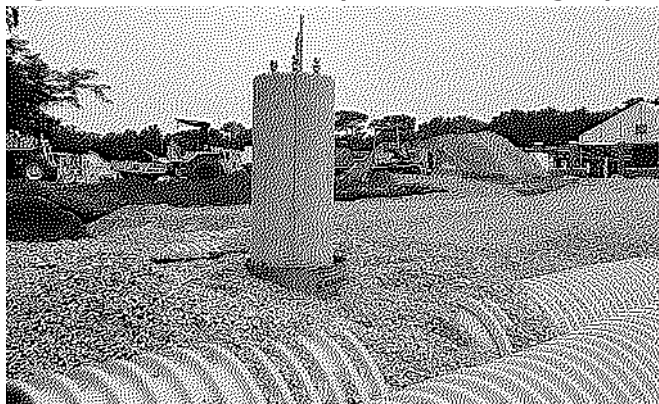
Figure 13 - Chamber bed placed around light post.
