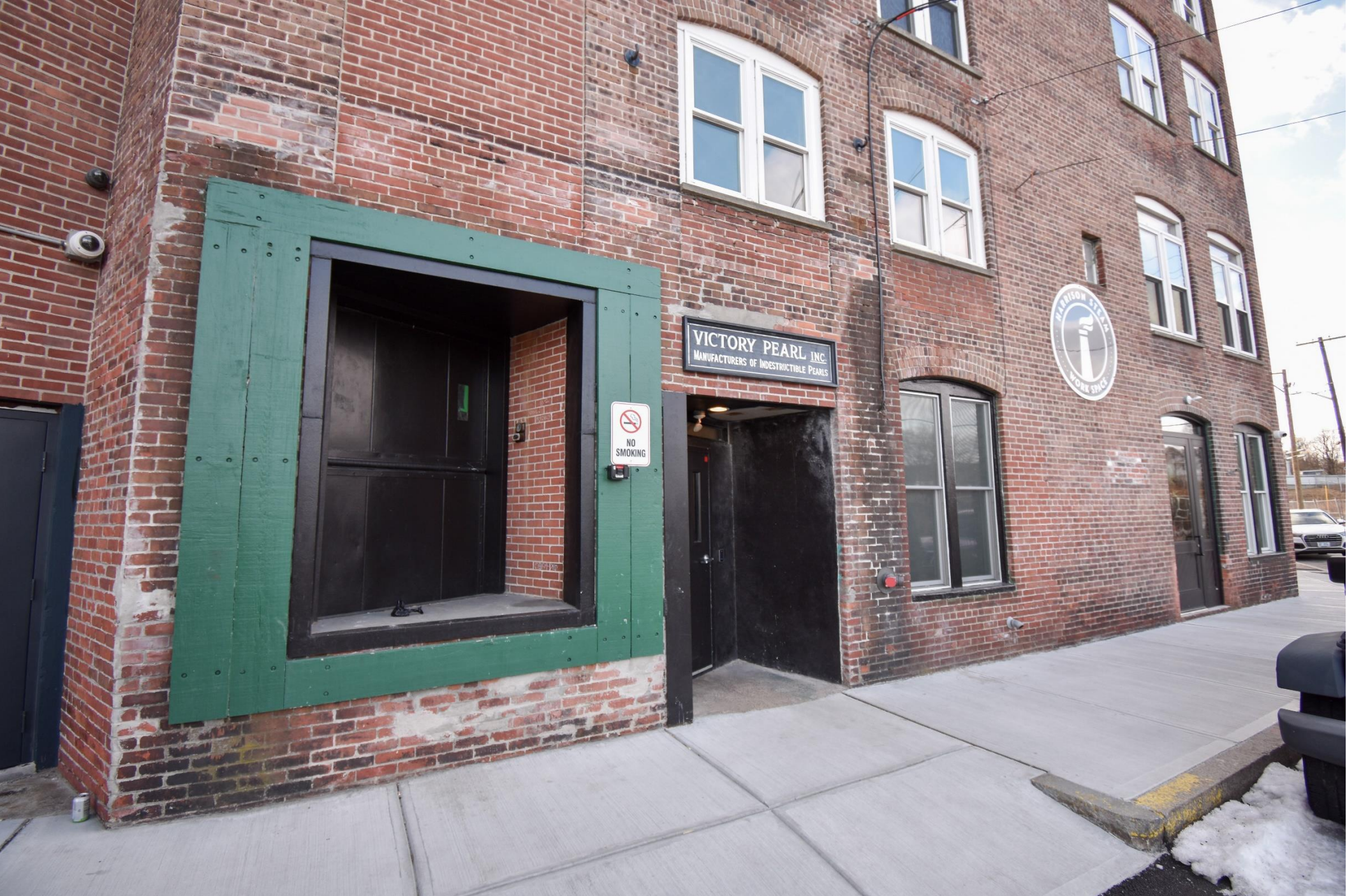
Photo 8. Elevator loading dock and entrances at Addition 2 (Addition 4 visible at far left), view southeast.
