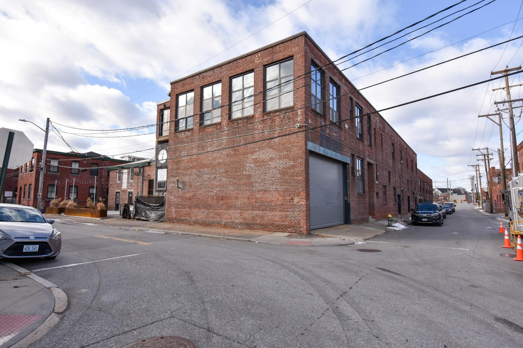
Photo 9. Streetscape from corner of Dike and Troy Streets showing (L-R) (43 Troy Street on the far left) Addition 1, Main Mill (loading/rigging dock), Addition 3, Addition 4, view southwest.
