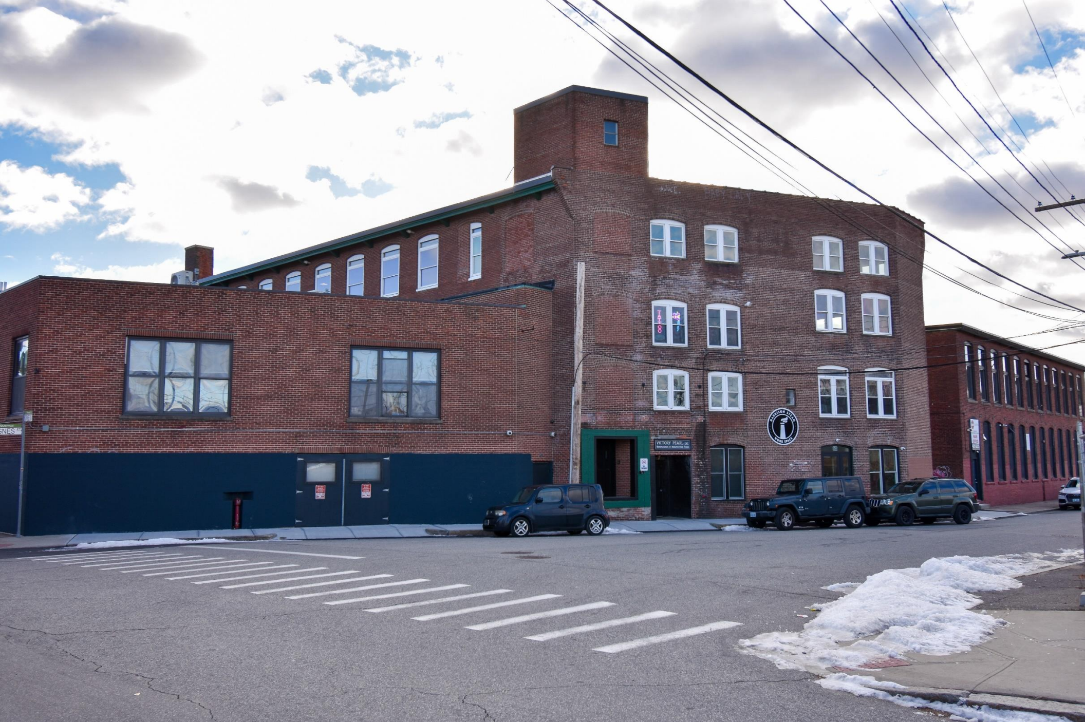
Photo 7. Streetscape from corner of Dike and Troy Streets with (L-R) Addition 4, Main Mill (fourth floor) and Addition 2, view southeast
