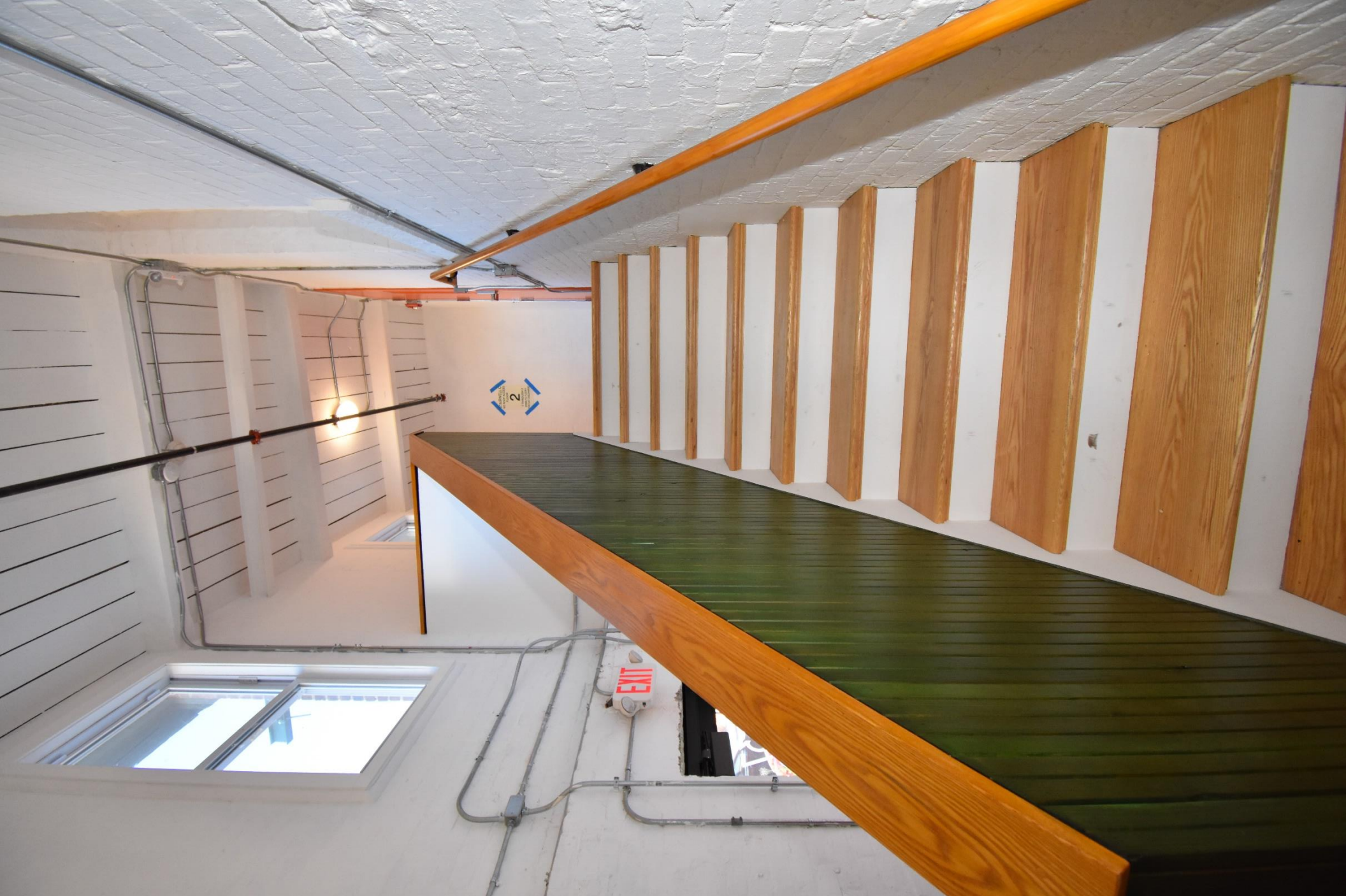
Photo 15. Interior of Addition 1 (first floor), view south.
