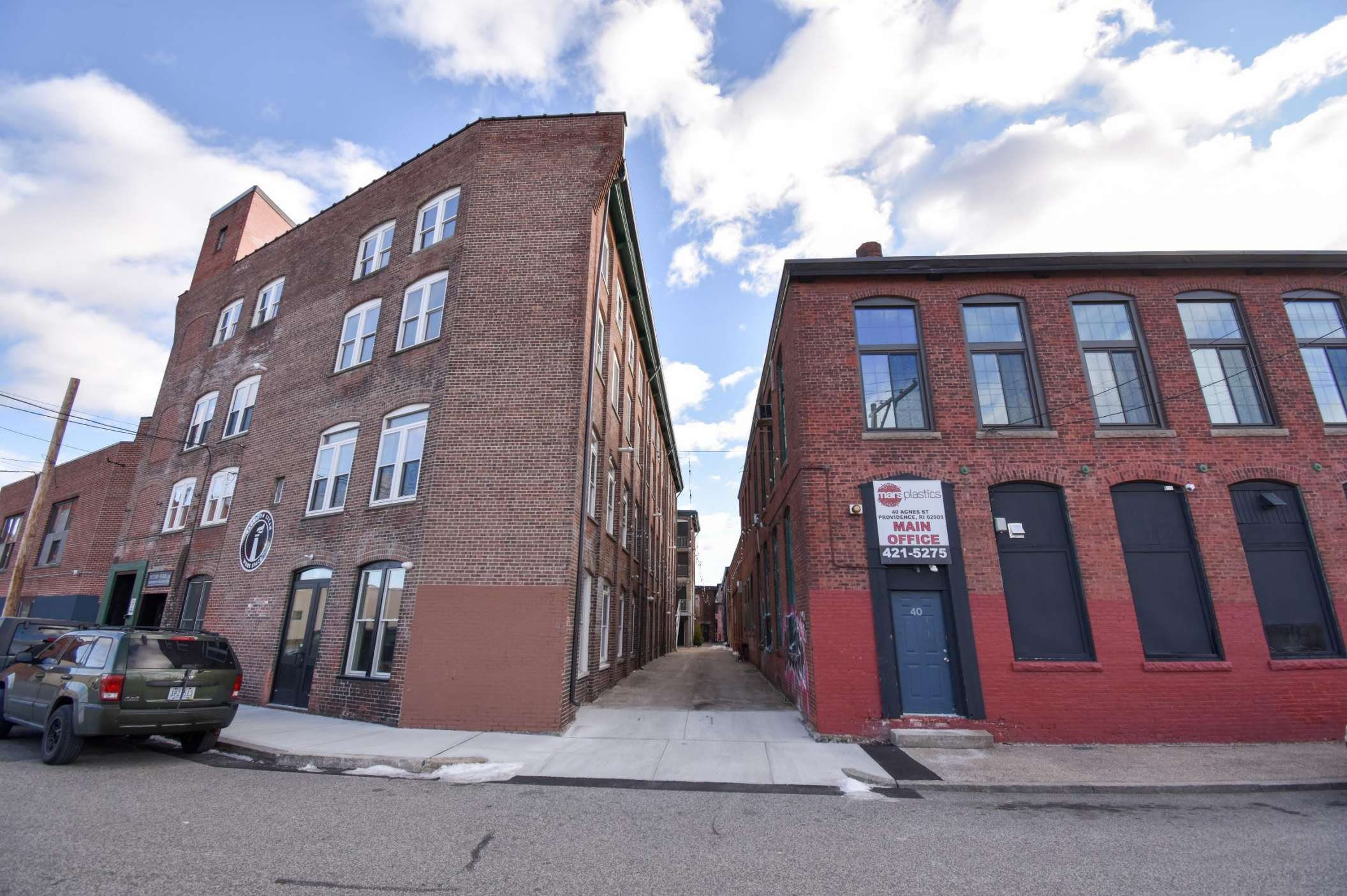
Photo 10. South alley from Agnes Street with (L – R) Addition 4, Addition 2, and First Engine/Boiler House (40 Agnes on right), view east
