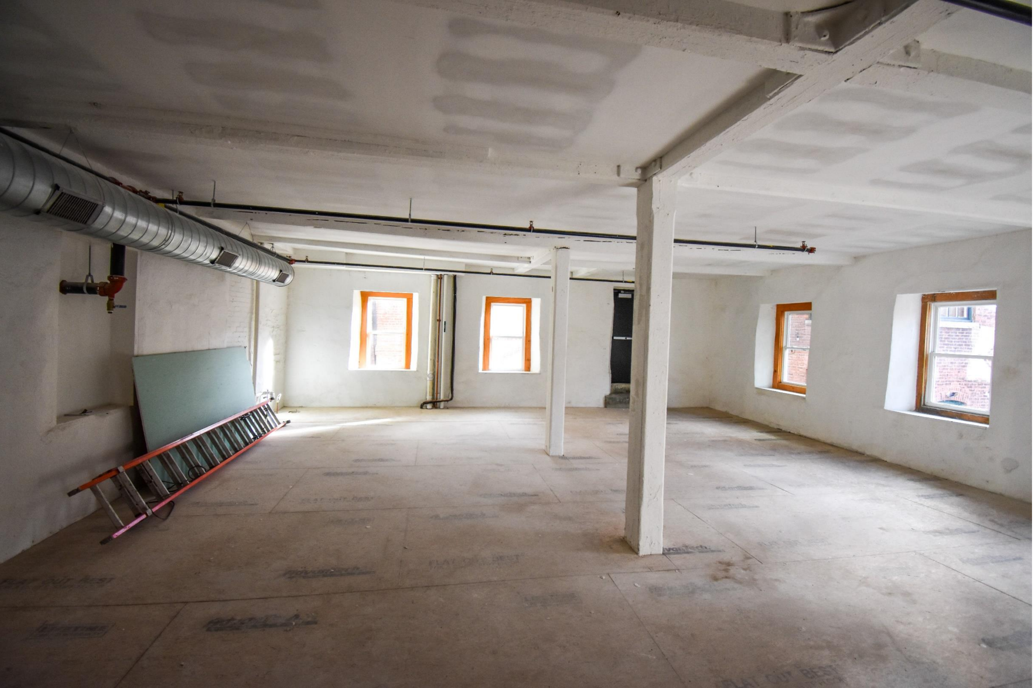
Photo 14. Interior of First Engine/Boiler House (second floor), view southeast
