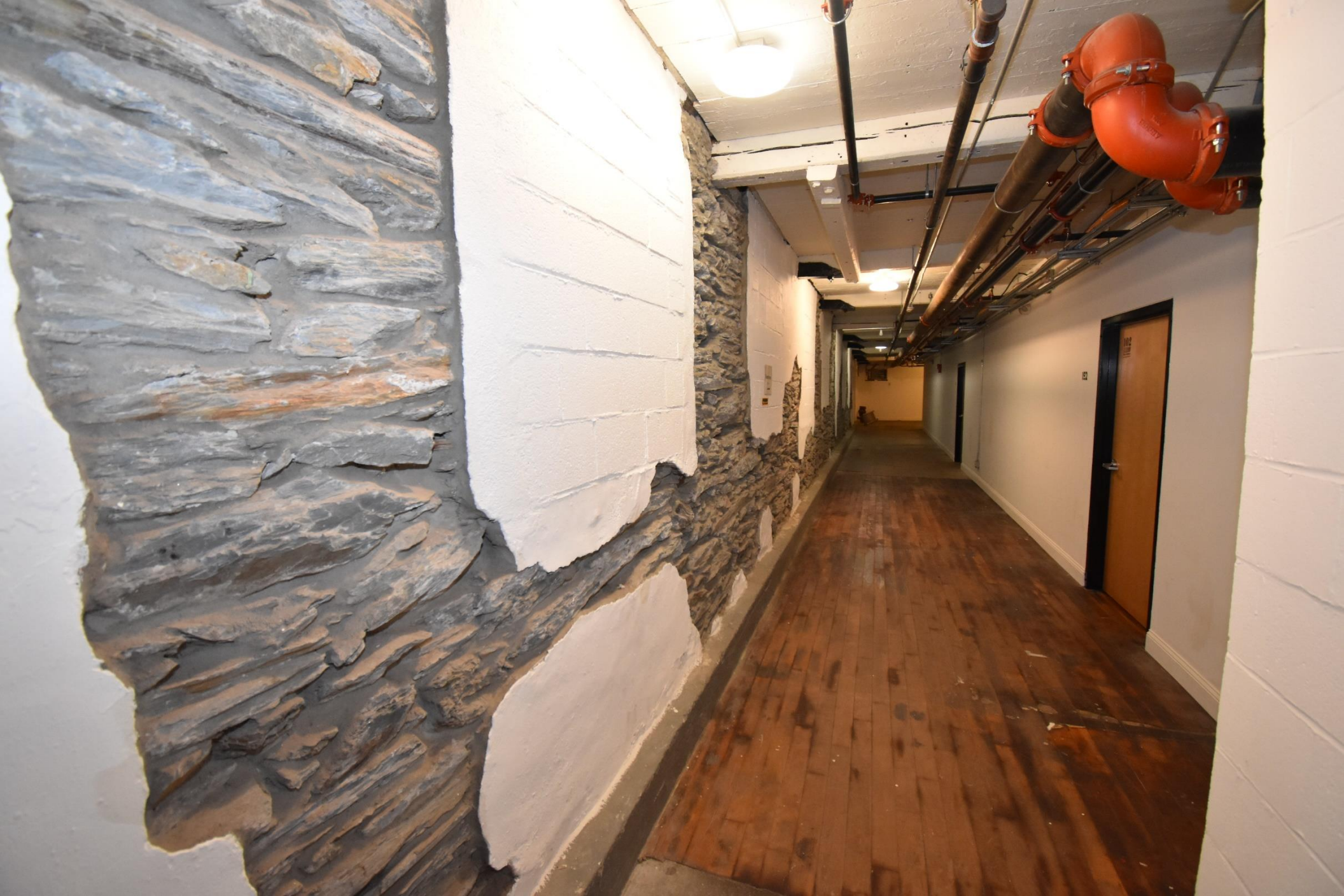
Photo 12. Interior of Main Mill's west wing (first floor), view east.
