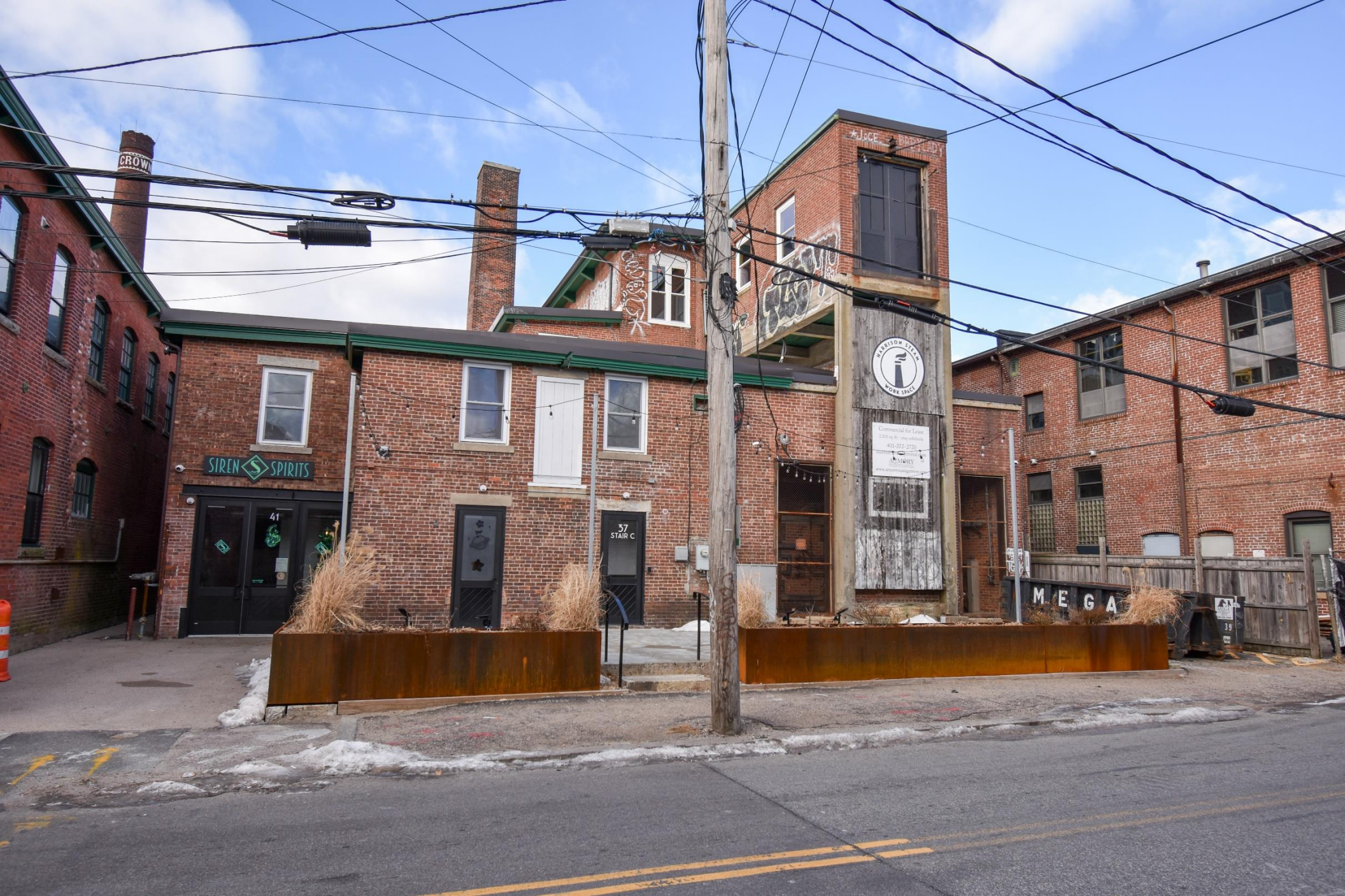
Photo 3. (L-R) (43 Troy Street on far left) South alley, Addition 1 with Chimney behind, fourth story of Main Mill with loading/rigging dock extension, Addition 4, view northwest.
