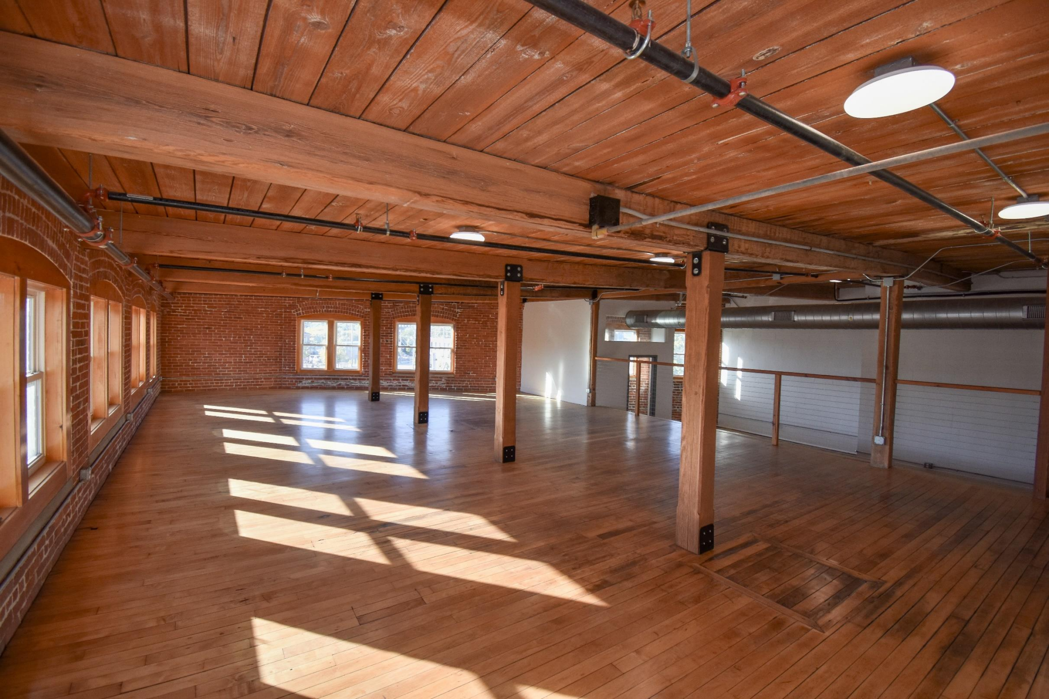
Photo 18. Interior of Addition 2 commercial unit (fourth floor), view northwest
