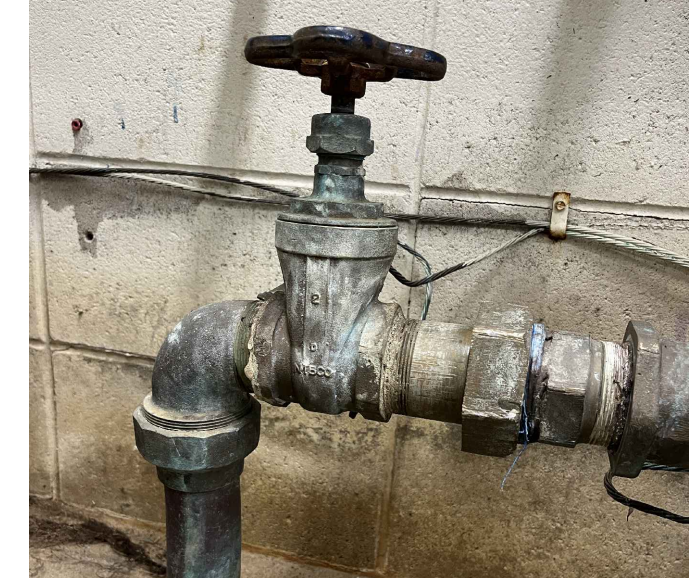
REMOVE AND REPLACE GATE VALVE WITH 2" BALL VALVE
