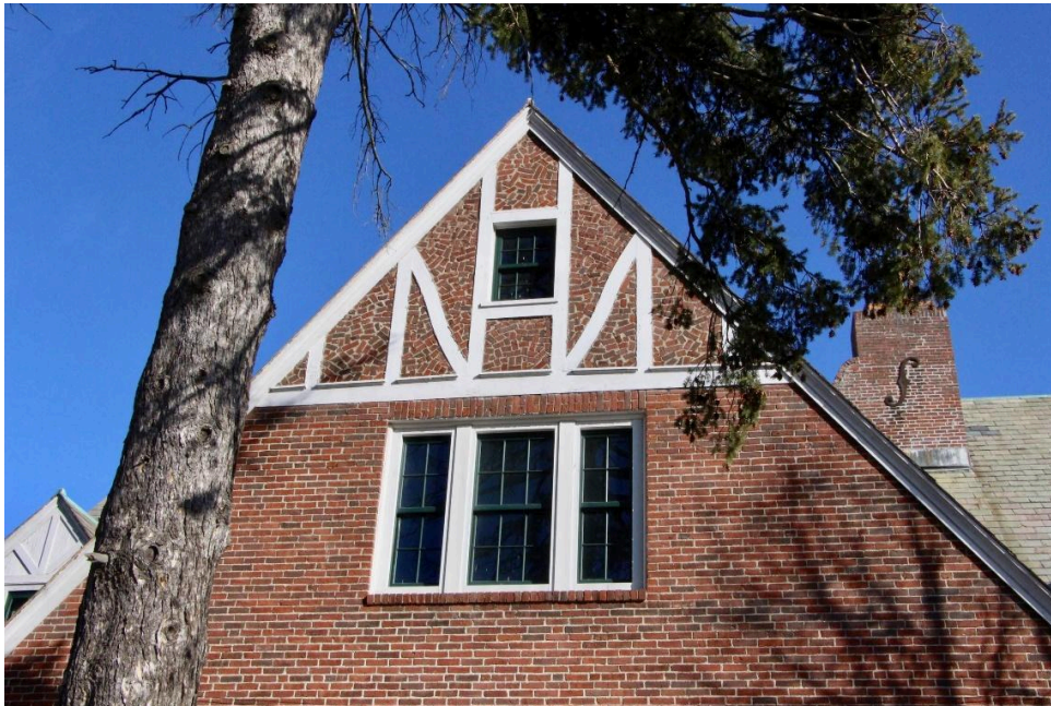
Figure 6: Example of uncoursed brickwork and decorative half-timbering in apex of cross gable.
