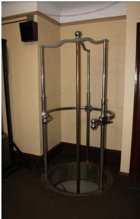
Figure 17. Fire pole in second-story dormitory/day room.
