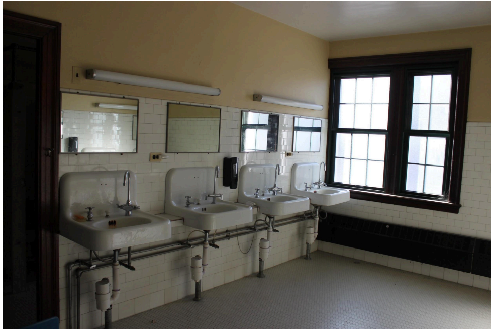
Figure 22. Historic fixtures in second story bathroom.
