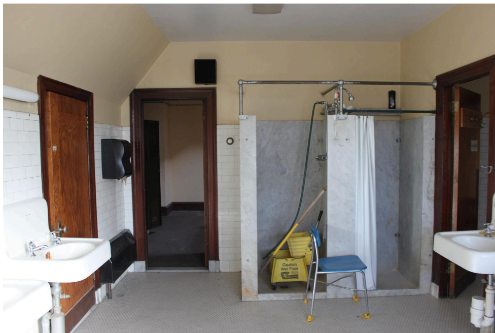
Figure 21. Historic fixtures in second story bathroom.
