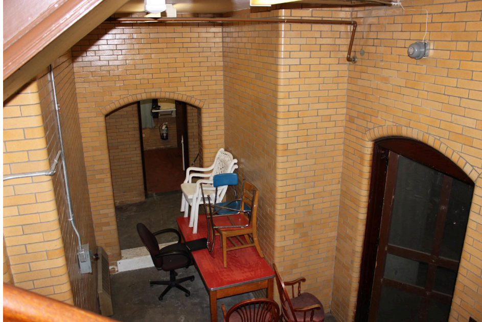
Figure 12. Looking west down from staircase to stairhall showing typical finishes and arched door openings.
