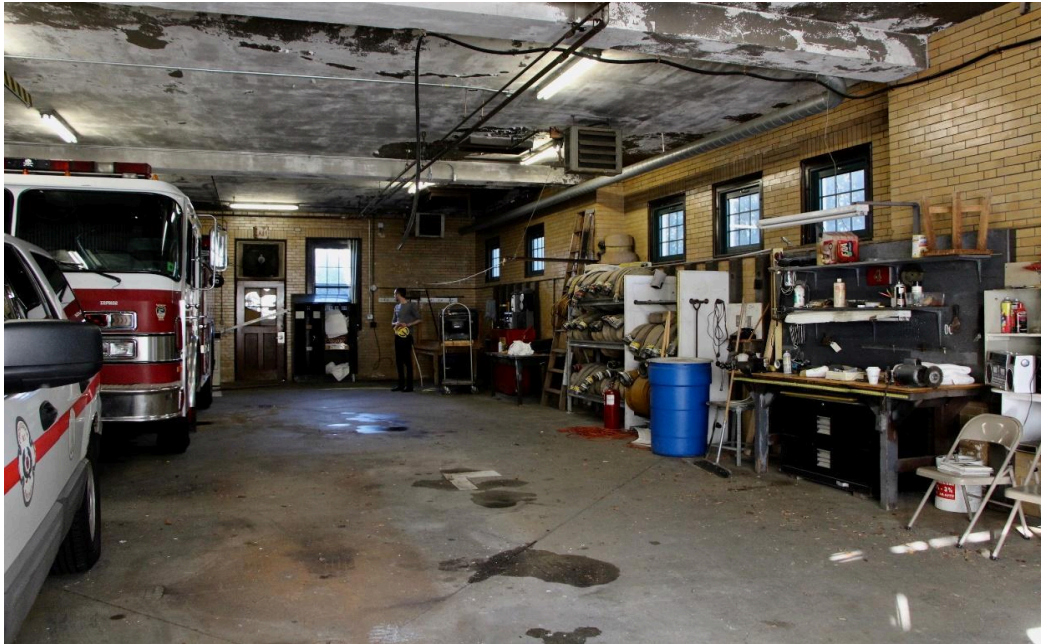
Figure 9. View of engine bay looking north.
