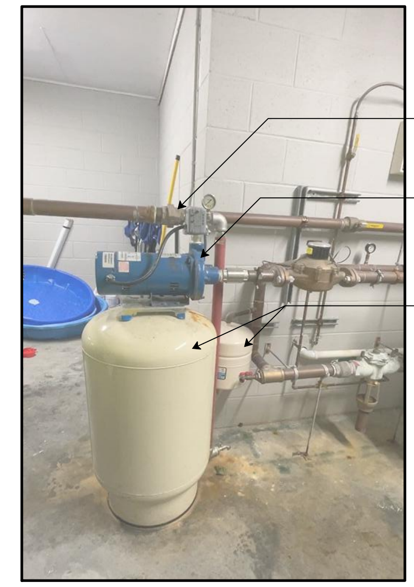
4 EXISTING BOOSTER PUMP AND TANK SYSTEM NTS
