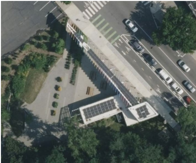
Figure 14. Existing on-site solar system at the Gateway
