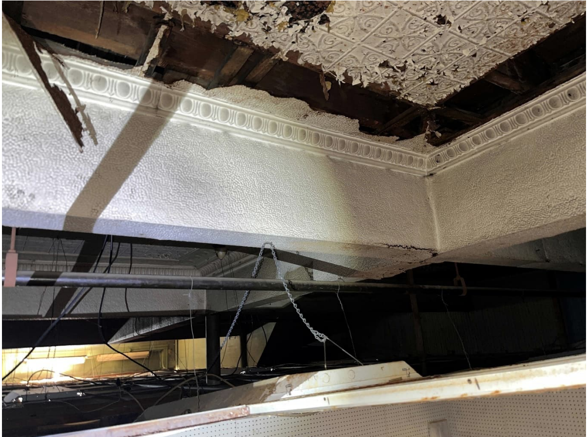
Photo 12 – Southern Portion, first story eastern half looking southwest. View of the typical structural beams and columns which support the wood framing of the second and third stories. This view is from above the existing drop ceiling. The column located in the center left provides support for the southeastern chambers above. Note the second story wood floor joists are visible through the deteriorated tin ceiling finish. Also note the deflection in the header beam above the eastern storefront window (background left – not easily discernable at this scale).
