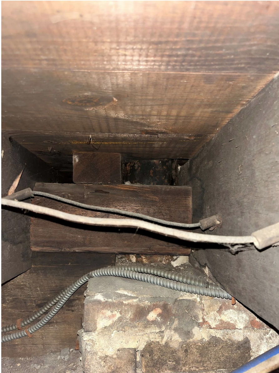
Photo 15 – Southern Portion, basement looking east. Photos shows the top of the CMU pier in the previous photo. The first story metal column is visible in the upper center-right of the photo (black/rust colored). The CMU pier also supports a large wooden beam (on the bottom left). The first story wood floor joists are visible on the left and right edges. The wood in the foreground adjacent to / in front of the metal column appears to be subfloor blocking.
