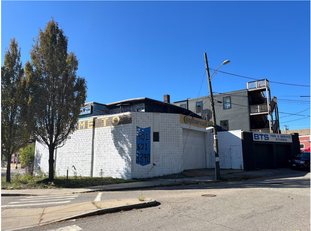
Photo 8 - 113 Broadway looking Southwest. The Eastern Portion of the building is in the foreground constructed of white CMU block, the Northern Portion is to the right (with the BTS sign), and the Southern portion is in the background. 117 Broadway is the green building with multiple wood decks in the background.
