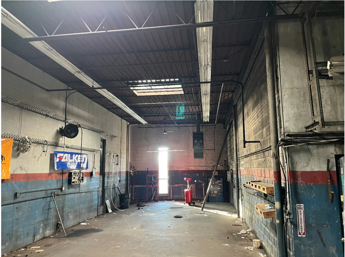
Photo 25 – Eastern Portion, typical interior view looking south. Note the typical construction – CMU block walls with open web steel joists spaced at 4' on center which support corrugated metal roof panels and membrane roofing. The CMU wall on the right side was constructed as part of the "southeast protrusion" - note the open web joists are supported on a steel header beam and steel columns which are completely independent of this older CMU wall.
