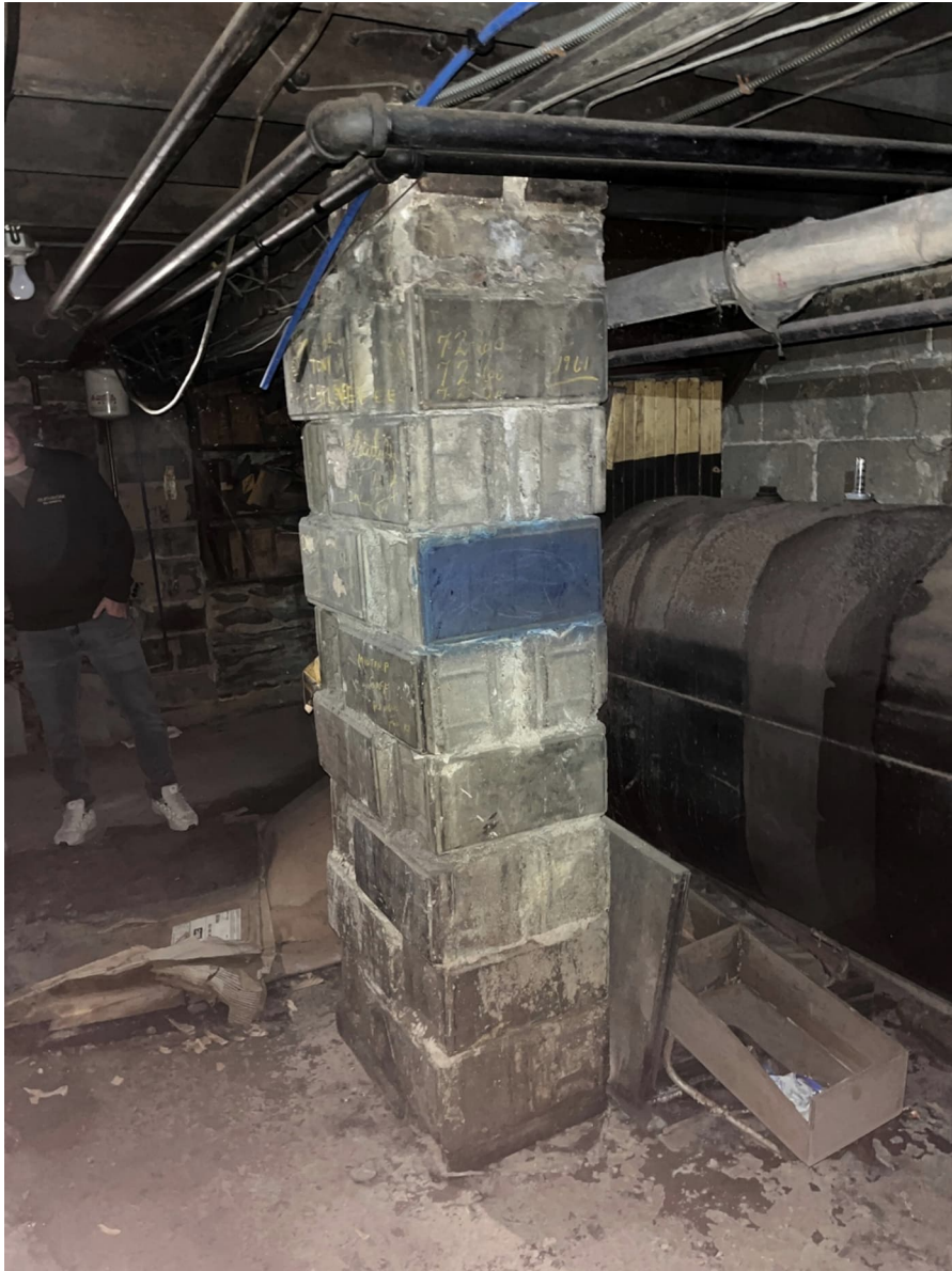
Photo 14 – Southern Portion, basement looking southeast. Typical CMU pier which supports a first story metal column. Note the CMU block is the same as those utilized for the eastern exterior wall and the Northern Portion exterior walls, which suggests they were constructed at the same time. The original rubble stone foundation wall is visible in the background as well as a CMU pier that has been integrated into the stone wall which supports one of the south façade storefront metal columns.
