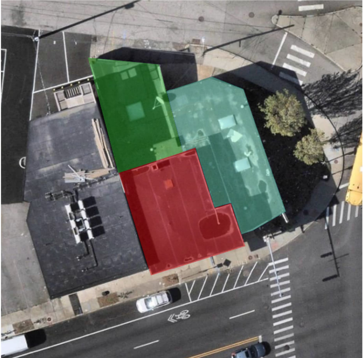
Photo 1: 113 Broadway Building Overview. Red = Southern Portion, Green = Northern Portion, Cyan = Eastern Portion. Note large puddle on roof of Southern Portion. This is the location of the “southeastern protrusion” noted in the report.
