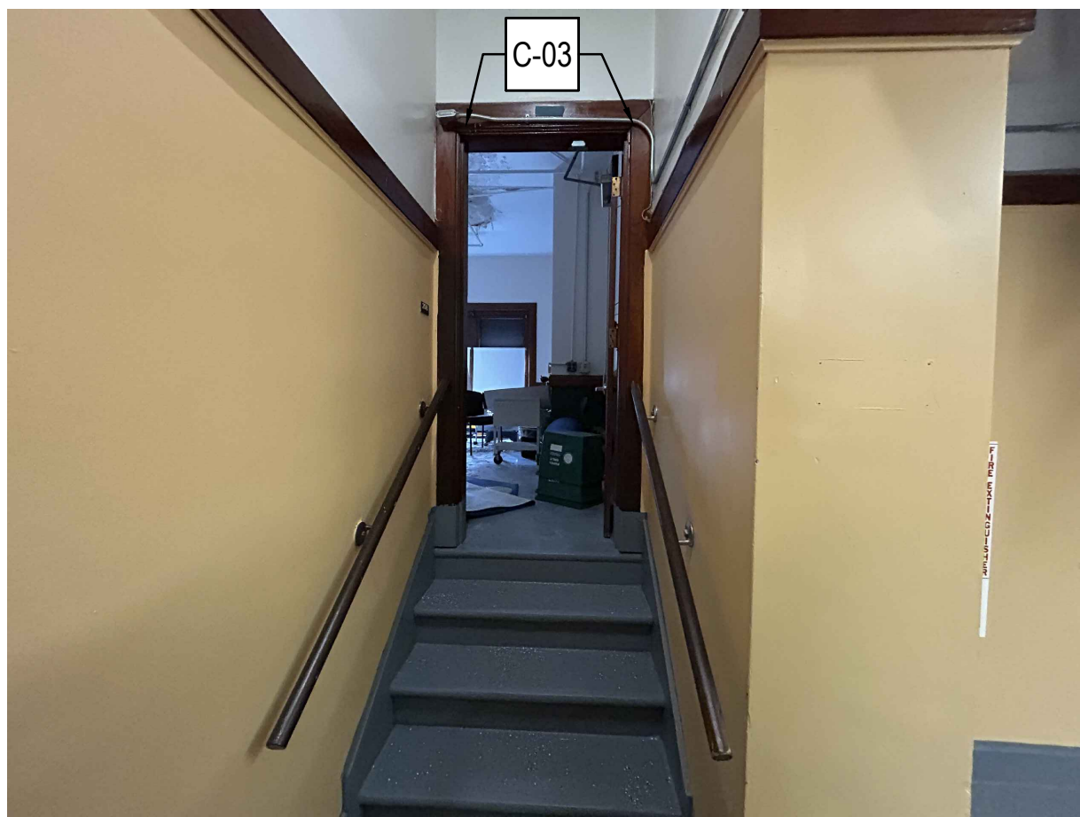
3 EXISTING ENTRANCE - OFFICE
