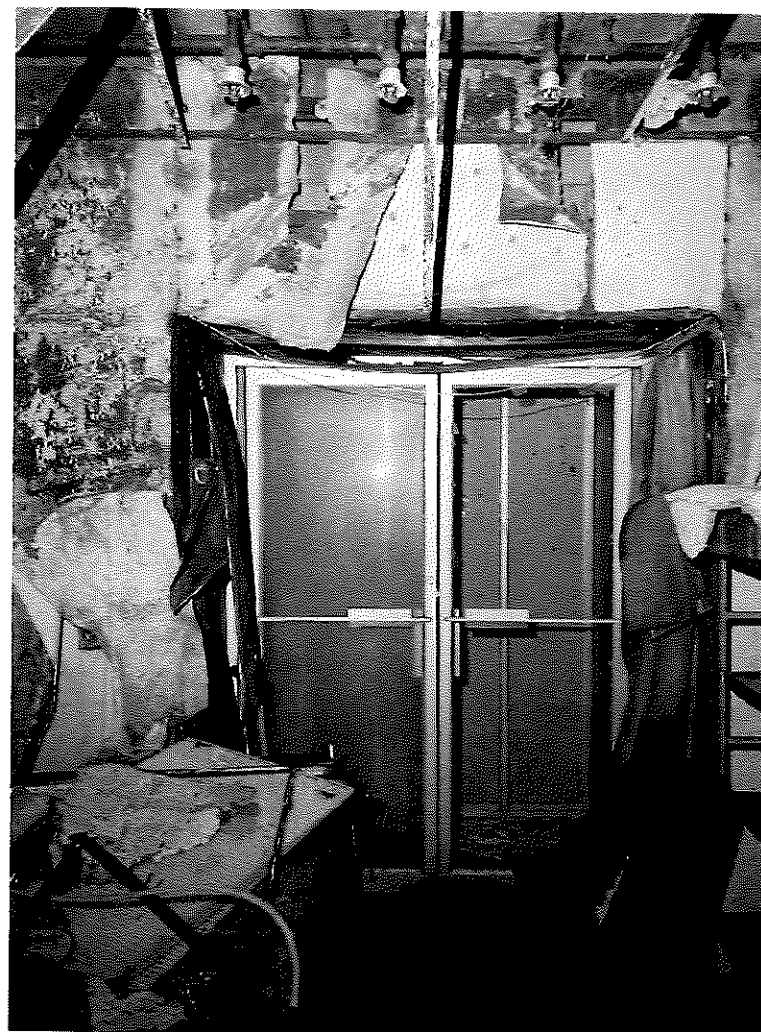
014: Aluminum door walled off to TAPA Building.
