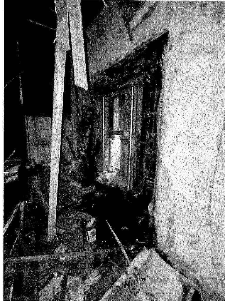
012: Bridge Interior conditions
