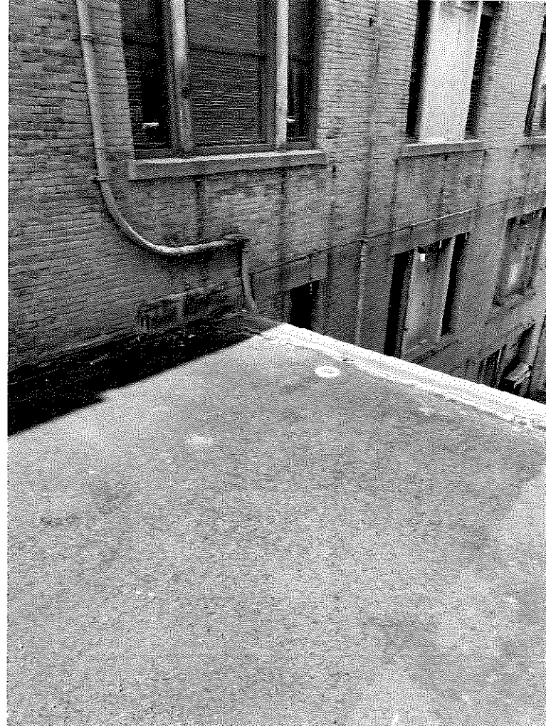
007: Roof conditions – Looking west
