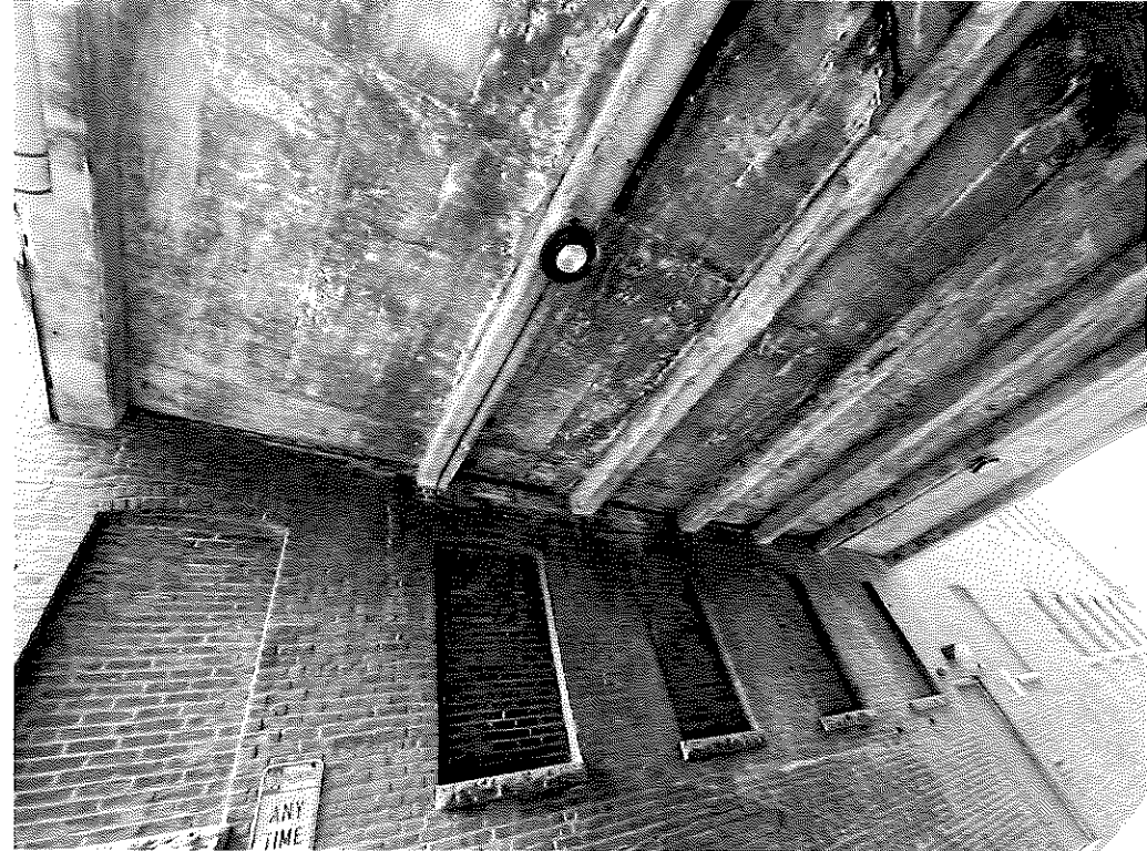
004: Clemence St. – Underside of connector Bridge
