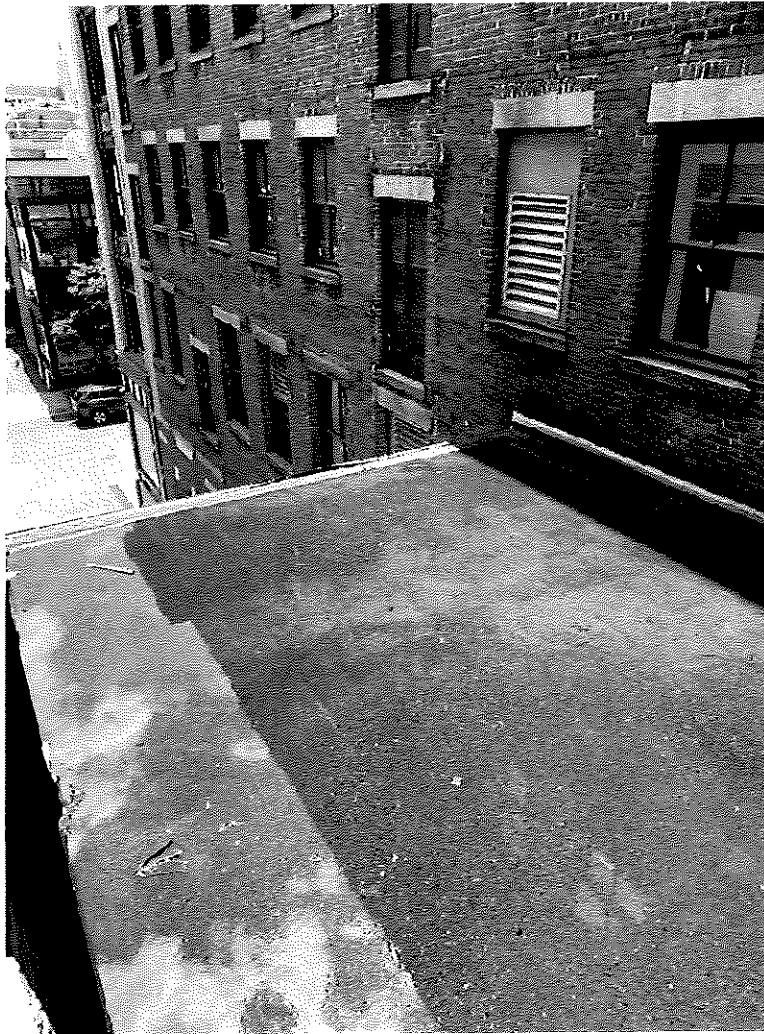
008: Roof. – Looking east
