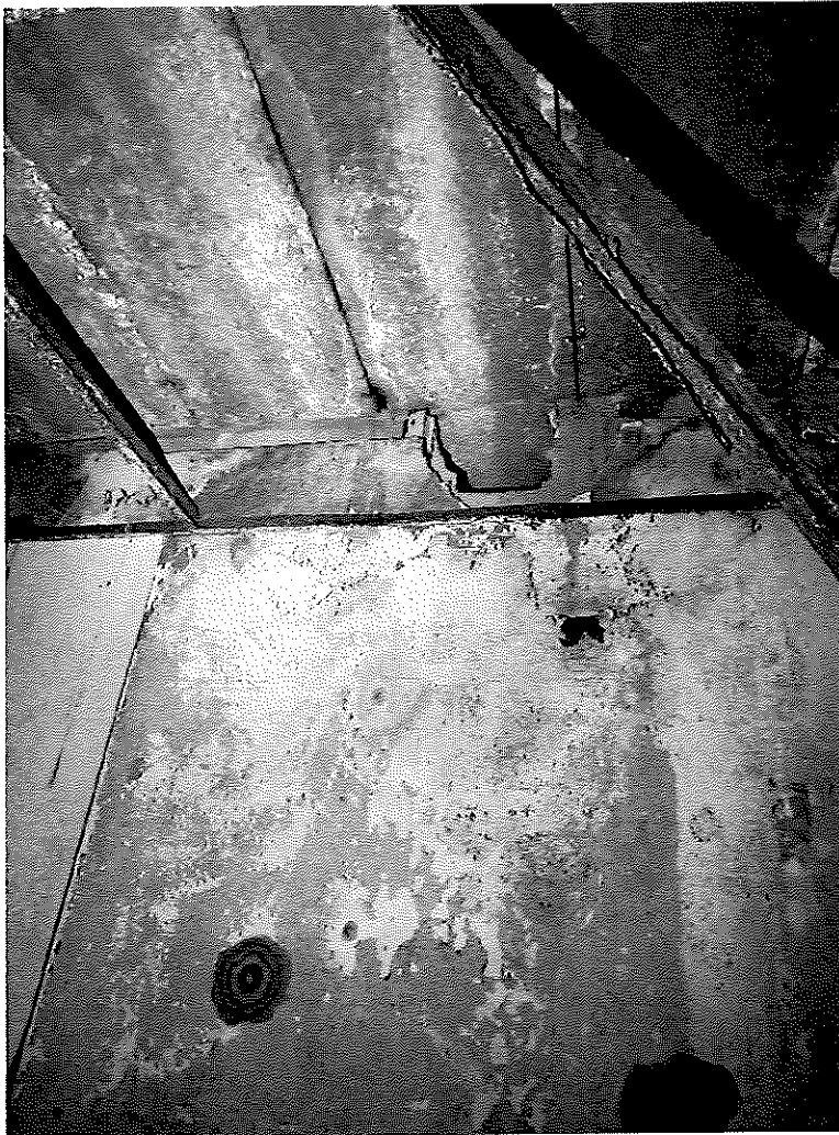
013: Image of precast concrete roof planks
