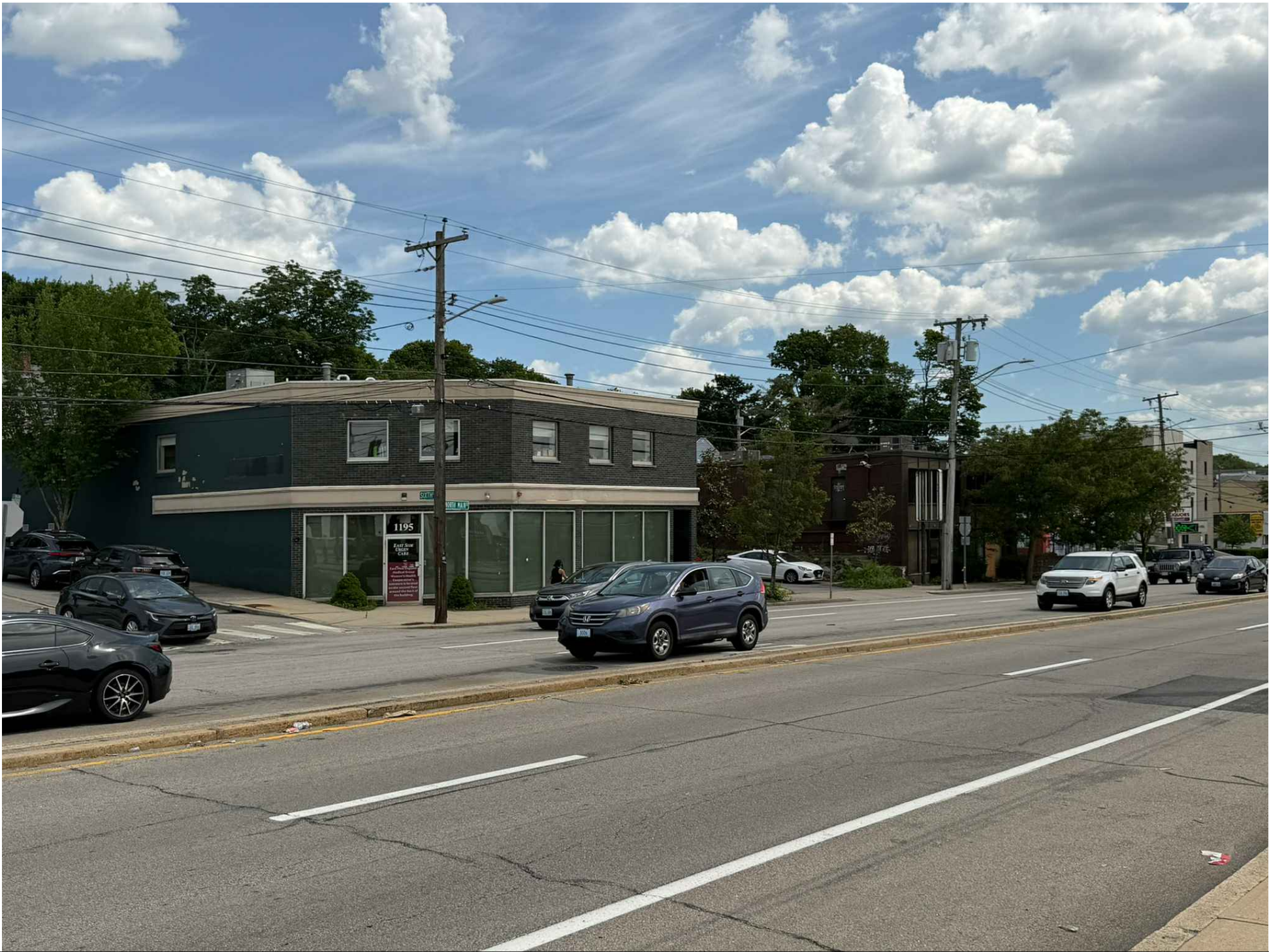
EXISTING EXTERIOR VIEW 1 - LOOKING SOUTHEAST ACROSS NORTH MAIN STREET
